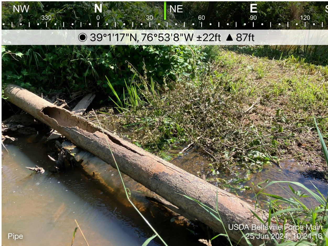
39 Figure 1.1 Exposed and damaged sewer pipe within stream. Source: Wetland Studies and 40 Solutions, Inc.
