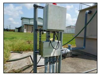
Photo 43. View of electrical panel/control box associated with the sewer treatment plant.
