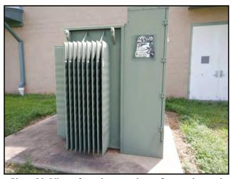
Photo 29. View of a pad mounted transformer observed on the central eastern portion of the Subject Property.
