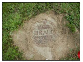
Photo 51: View of a drain manhole observe don the southeastern portion of the Subject Property.
