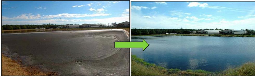
**FIGURE 8** | Swine lagoon conversion into aerobic pond. Picture on the left shows Lagoon 1 under traditional management before start of the project, and picture on the right shows the same lagoon after the wastewater treatment plant (background) was in operation for about 10 months.
