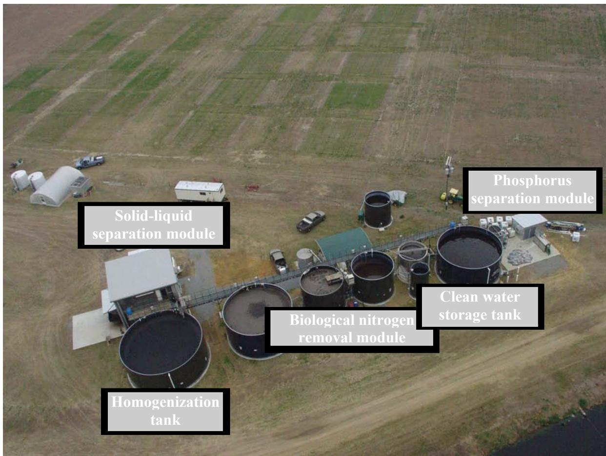
**Figure 3. Full-scale wastewater treatment system that replaced the swine lagoon.**
