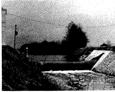
Figure 2. The Fabridam, a patented structure by N.M. Imbertson and Associates, Inc., Burbank, California, designed to Agricultural Research Service specification and put into operation across Mitchell Creek on April 2, 1982.
