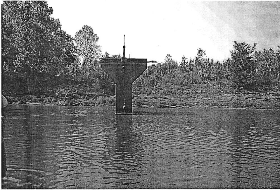
Figure 4. Photograph of principal spillway and earthen embankment at Hubbard-Murphree reservoir (September 2000). Note that the principal spillway is in disrepair and that the current water level is well below the designed stage.
