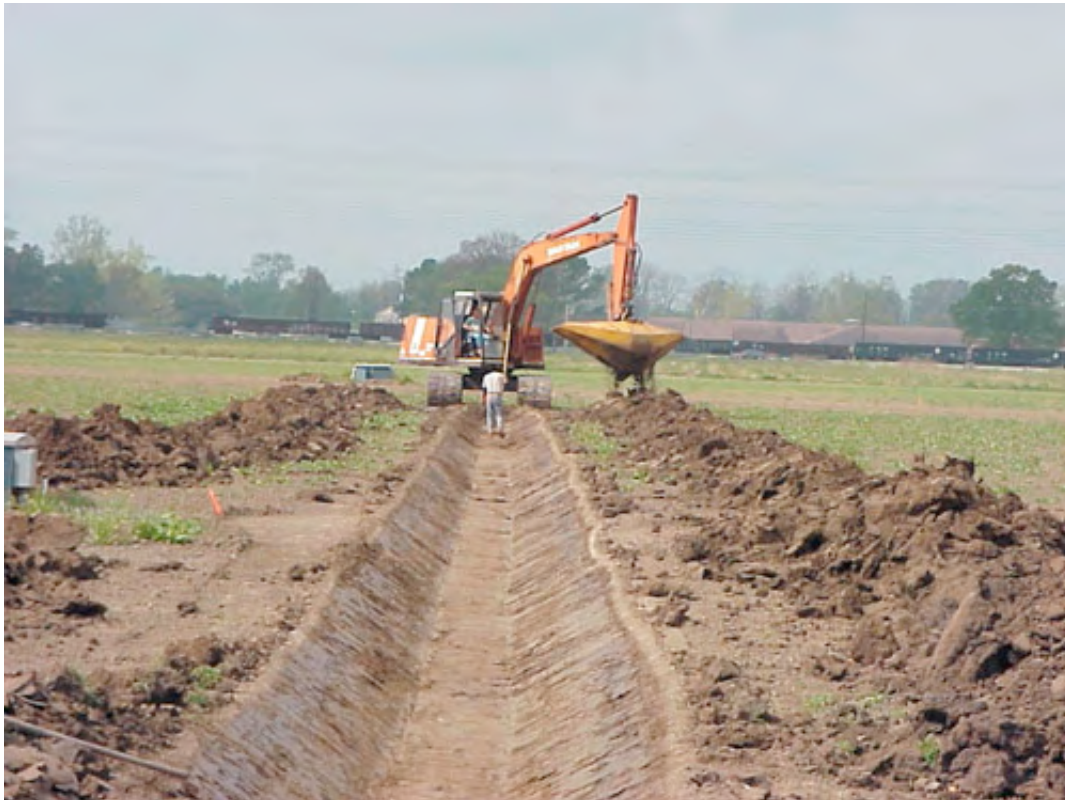
Construction of surface drainage ditch systems for runoff waters collection
