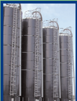
upright: oxygen-limiting glass-lined
