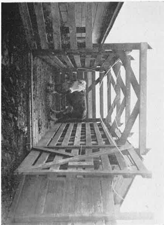
Figure 28.—Scales with rack for weighing steers. The gates are operated from the outside by means of the ropes and pulleys. The gate automatically locks by means of a spring catch. May 28, 1941.
