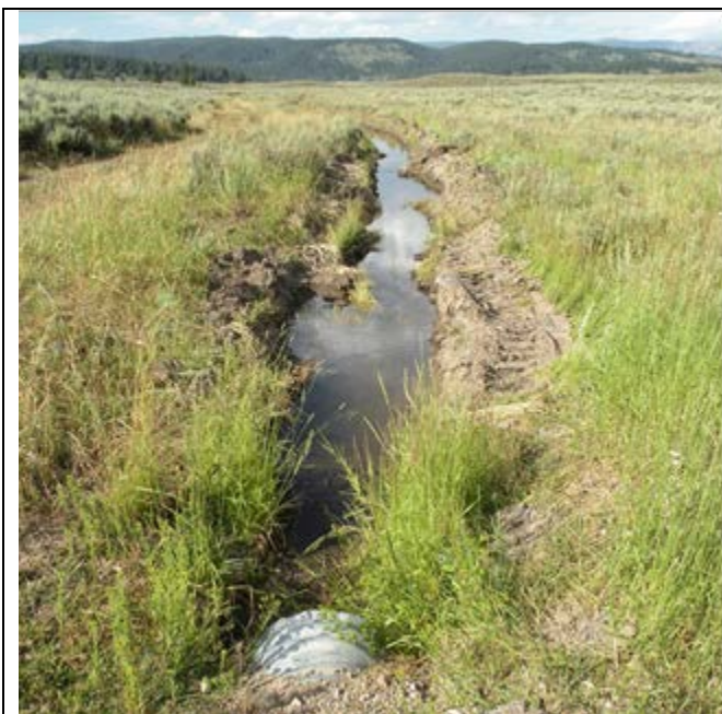
Figure 34. Ditching and Maintenance, Henninger Ranch
