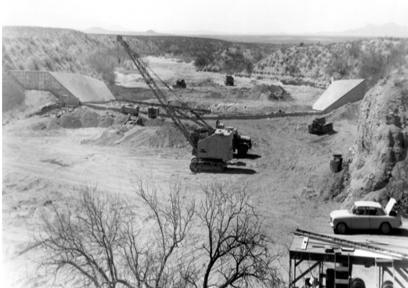
Construction of Flume 1, 1964.
