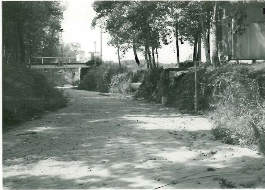
Figure 2.--Section of stream channel with recorder shelter on right bank. Gage well and stream-gaging section are shown in background.
