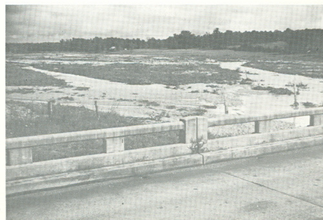
Figure 2. Sediment-plugged channel.
