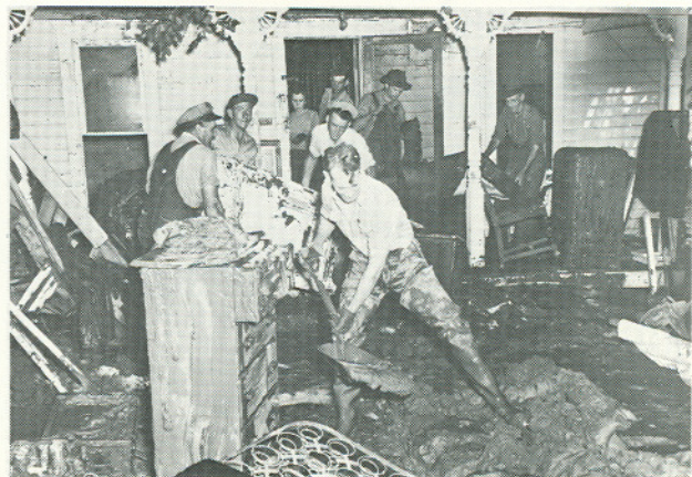
Figure 7. Home damaged by sediment.
