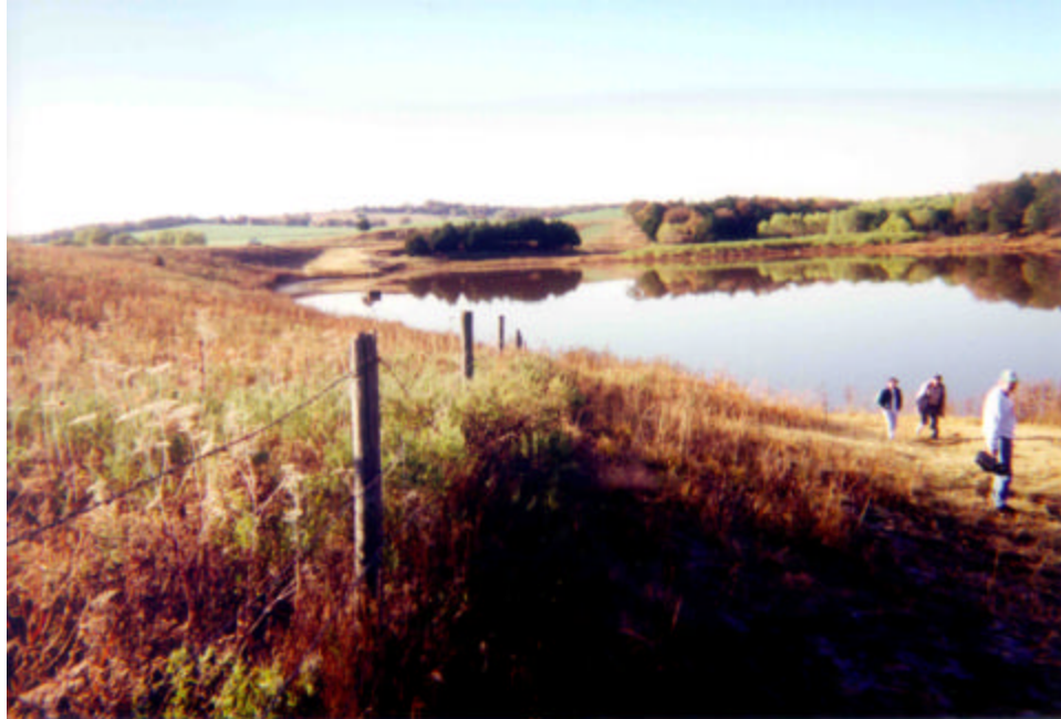
Figure 2-1. Photograph of Sugar Creek #12 looking directly south showing earthen embankment on left, spillway channel in far distance, and reservoir (November 1999).
