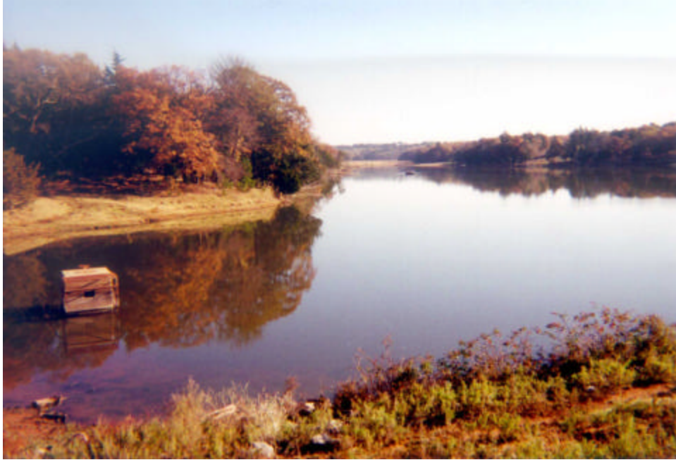
Figure 2-5. Photograph of Sugar Creek #14 looking northeast from the embankment showing reservoir, primary spillway drain on left, and main tributary source in far distance (November 1999).
