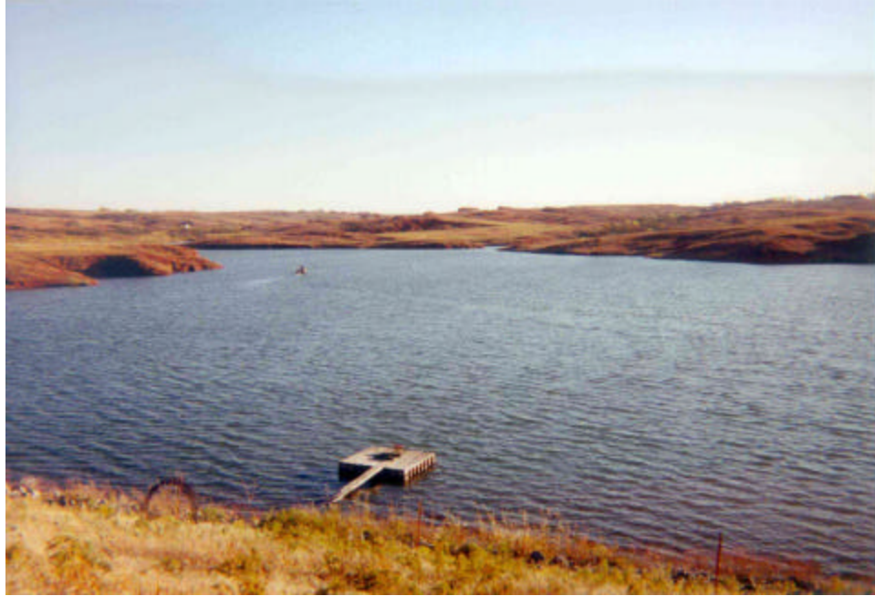
Figure 2-8. Photograph of Sergeant Major #4 looking almost directly south from the embankment showing reservoir, primary spillway drain in foreground, and the vessel used during seismic surveying in the distance (November 1999).
