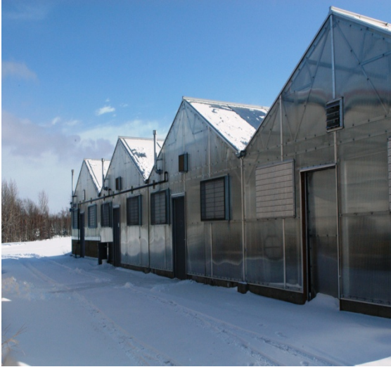
Looking Northeast at the four Palmer ASPGB greenhouses in February.
