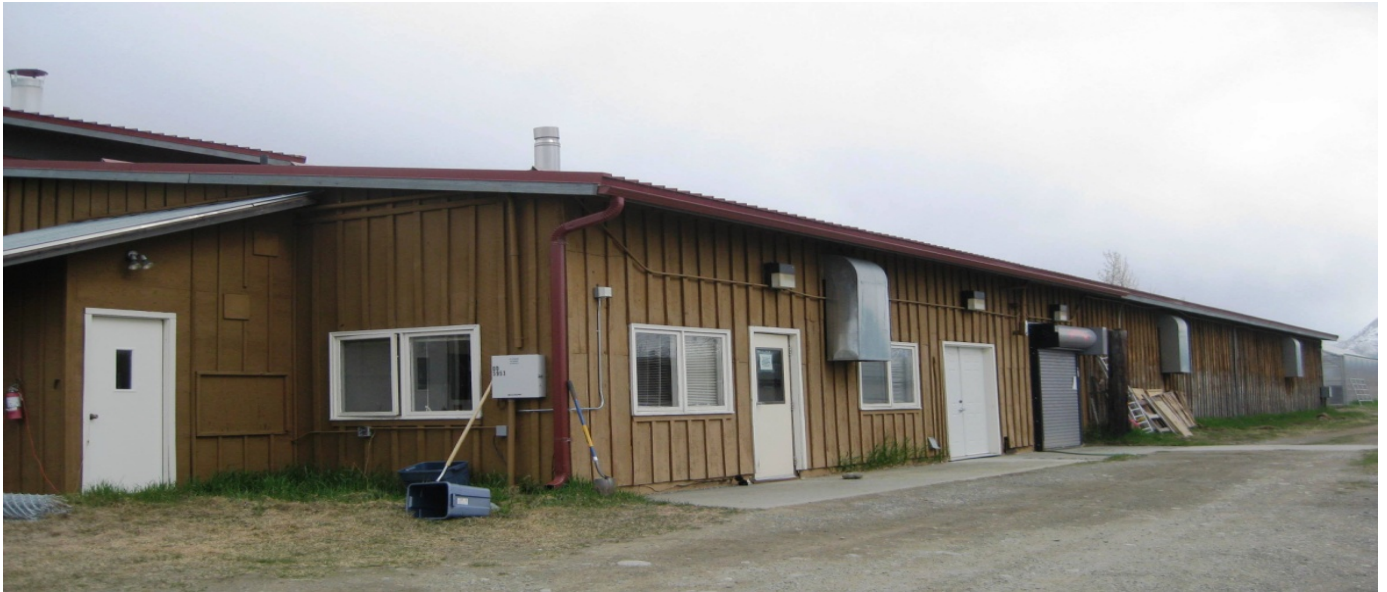
Front of ASPGB building looking East at the main entrance.
